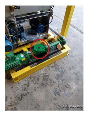
Project Area Sludge Inlet Connect DN50pipe from sludge holding tank to sludge feed pump.
